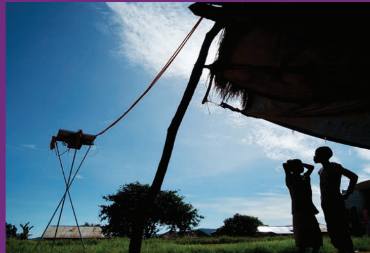
PHOTO: Wires connecting Devergy households / CREDIT: Devergy
