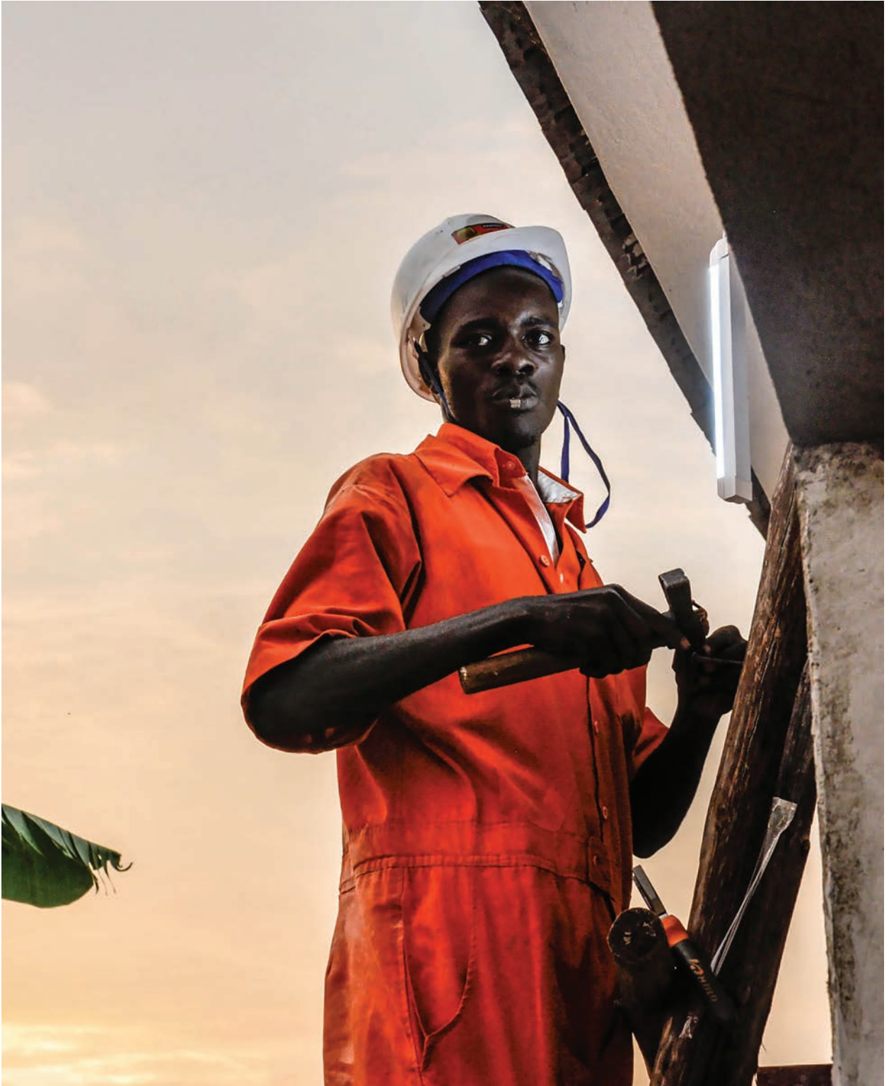
PHOTO: Installing panels for SolarNow customers / CREDIT: Nicolas Guillen
