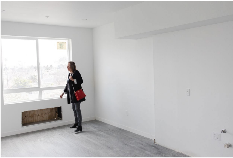
Deborah La Franchi at the apartment complex under construction in South Los Angeles.
